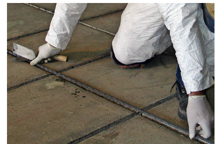
Near-Surface-Mounted FRP Reinforcement
