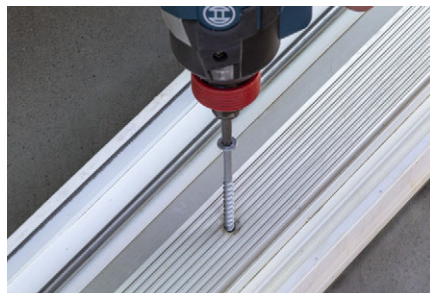
Sliding door track installation
