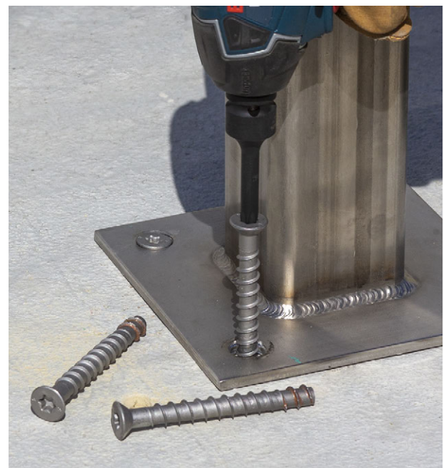
Titen HD Countersunk Installation
