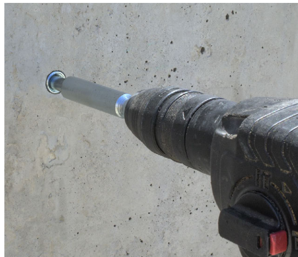
Anchor being set with SDS setting tool.
