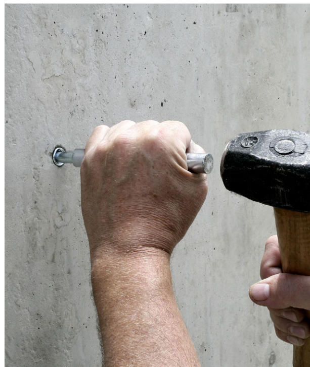
Anchor being set with hand setting tool.
