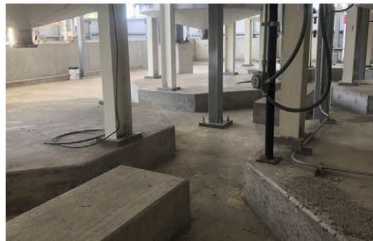
Typical medium-corrosive environment — exterior anchorage.
