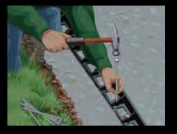
**6. EDGE RESTRAINTS** Install edge restraints as required. Pavers butting against curbs or foundations will not need an edge restraint. Various types of edging materials can be used. Nicolock recommends a Snap Edge edge restraint system since it is easy to install and will not rot or decay.
