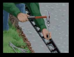
**6. EDGE RESTRAINTS** Install edge restraints as required. Pavers butting against curbs or
